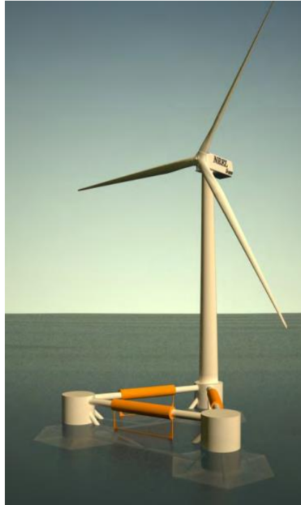
Figure 5.2.2.3: WindWave float with oscillating plates [29]
